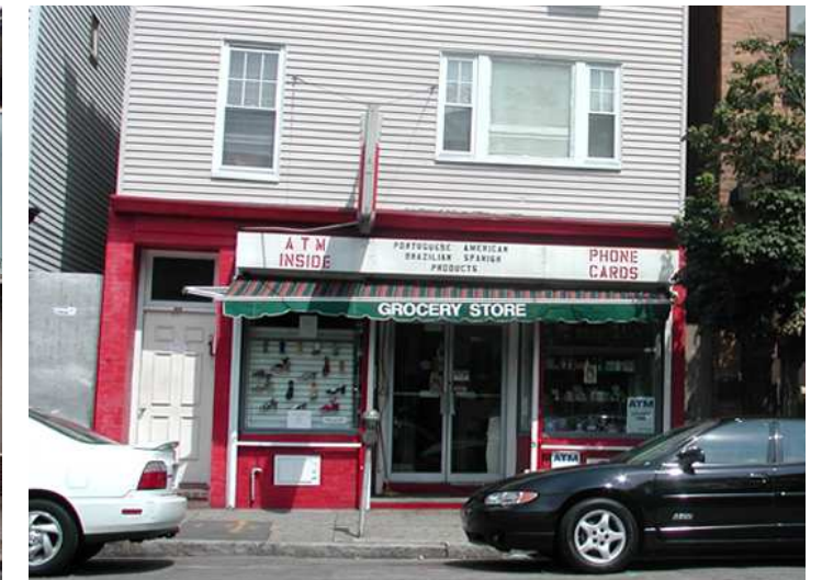
Pires Market: Existing Conditions
